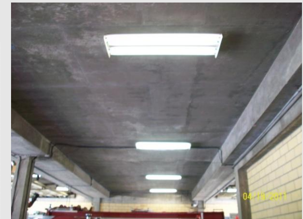
Lighting upgrade at Fire Station
