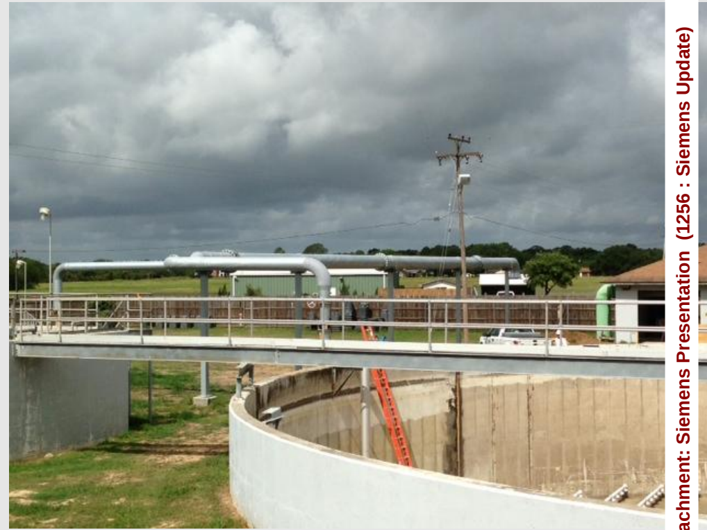
New Overhead Air Piping
