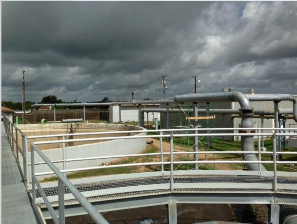
New Overhead Air Piping
