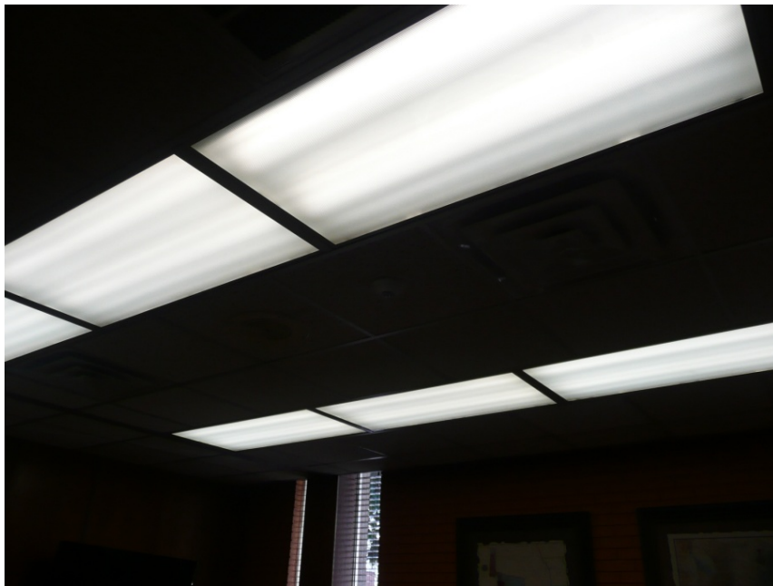
Figure 21: New Efficient T-8 Fluorescent Lamps (Conference Room)
