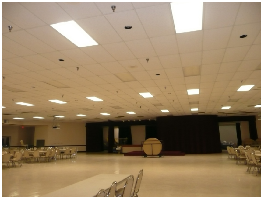
Figure 23: New Efficient T-8 Fluorescent Lamps (Banquet Room)
