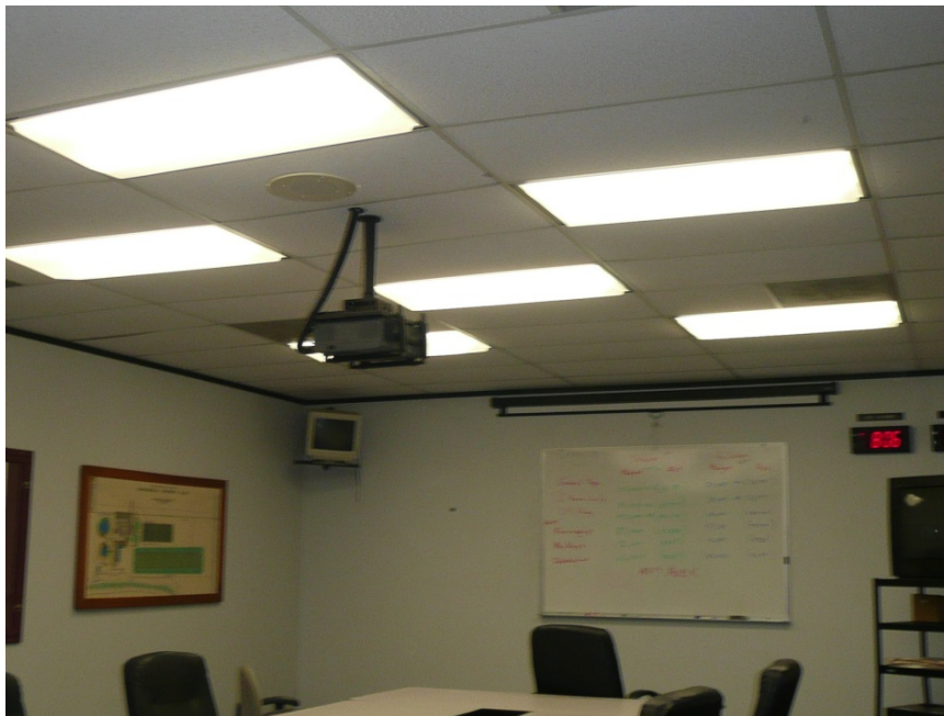
Figure 25: New Efficient T-8 Fluorescent Lamps (Conference Room)
