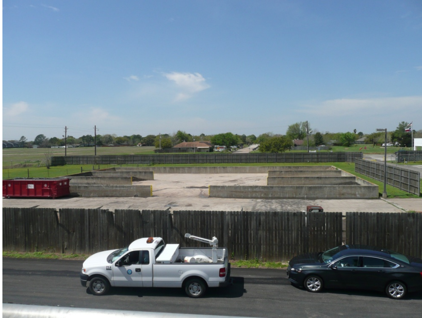
Figure 11: Drying Beds (Alternate View)
