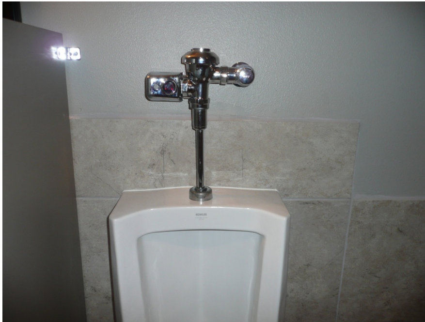
Figure 29: New 1.25 gpf Flush Valve Installed on Urinal (Men's Restroom)
