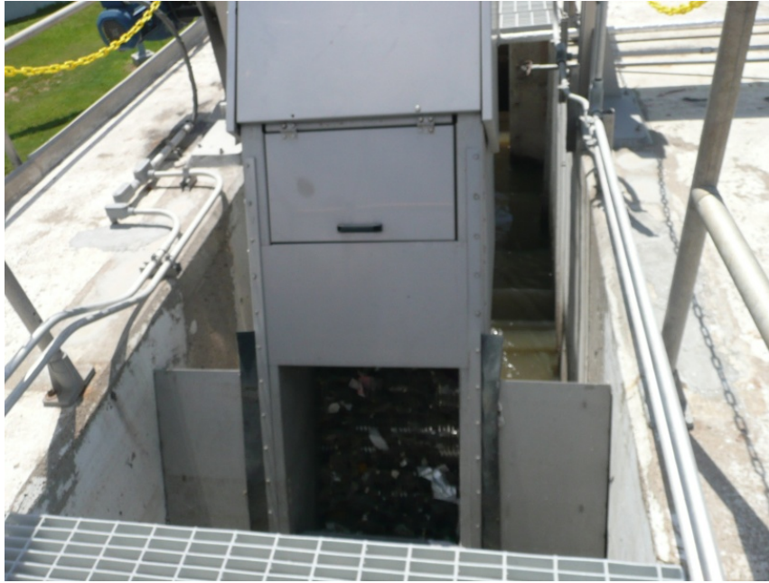
Figure 8: New JDV Fine Step Mechanical Head Screen (Headworks)
